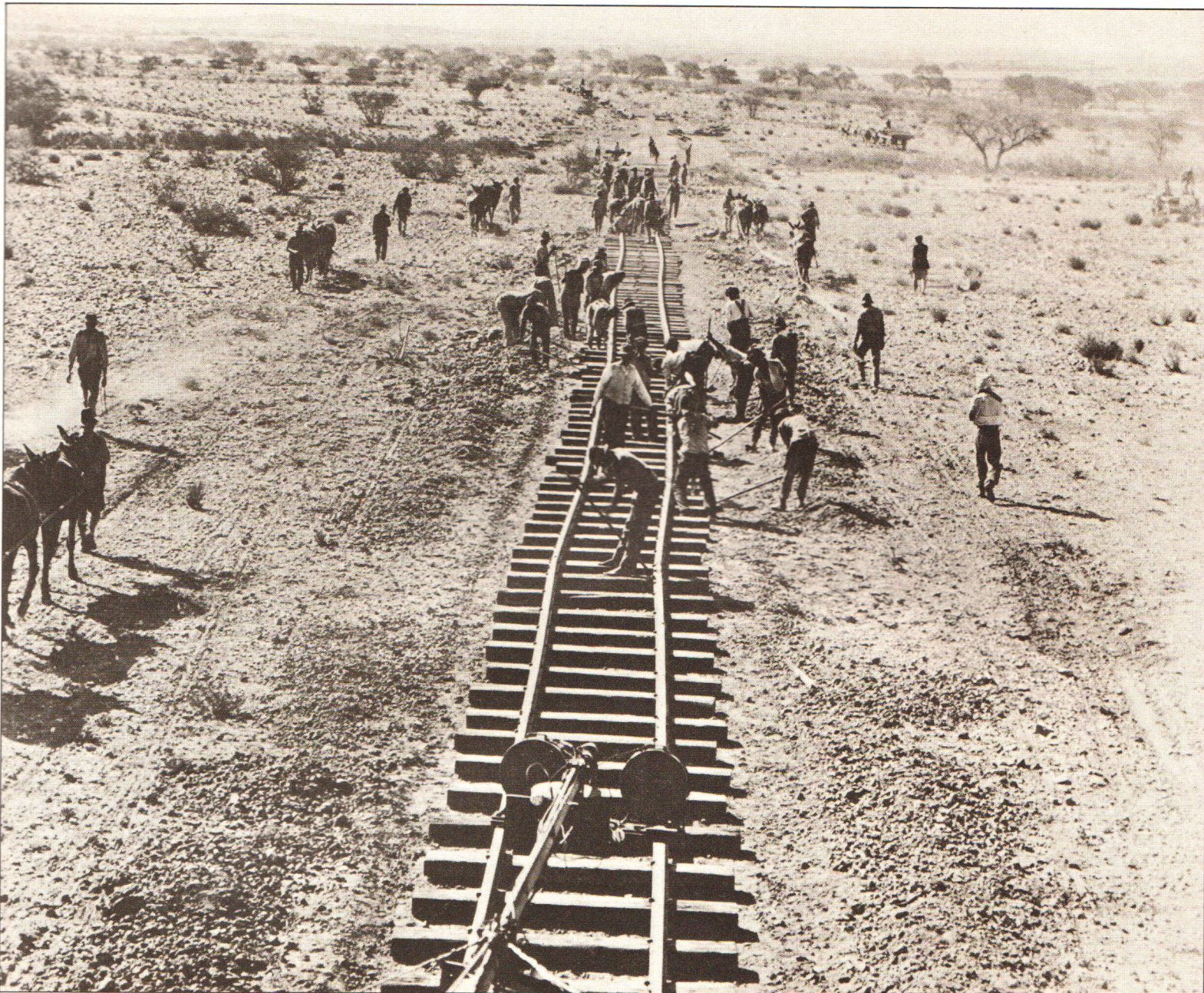
General Botha's men, eager to use the enemy's own rail-lines against them, re-lay the metals and sleepers torn up by the retreating Germans.
